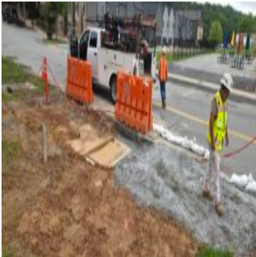
backfilled gab
