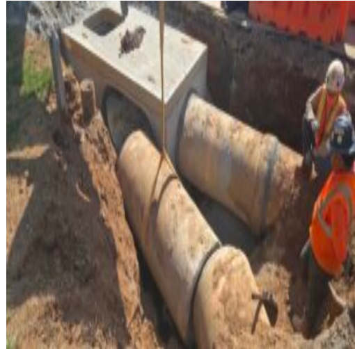
previous visit picture of the structure
