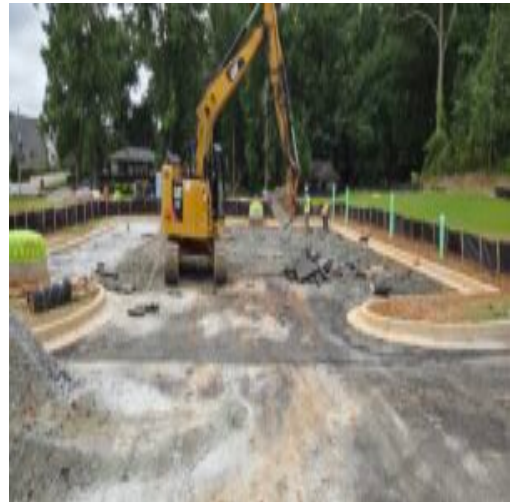
removing asphalt
