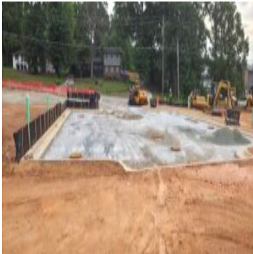
bad area fixed by contractor
