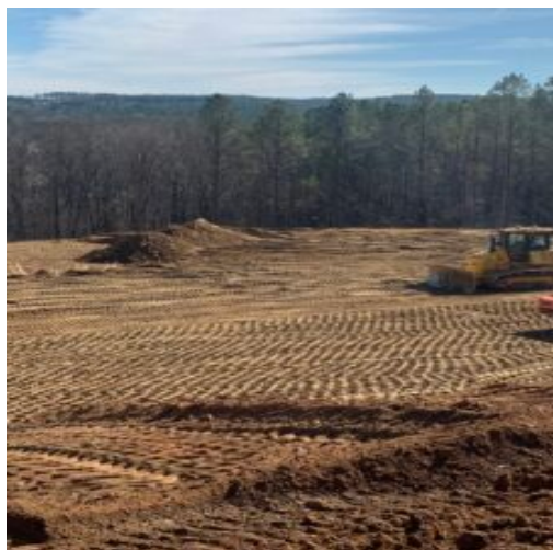
Fill placement at slope embankment
