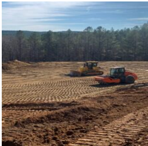
Fill placement at slope embankment
