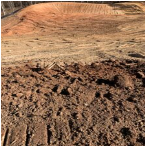
Fill placement at slope embankment ,topsoil and structural fill .
