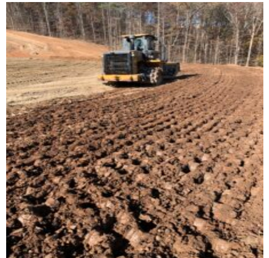
Fill placement at slope embankment ,topsoil and structural fill .
