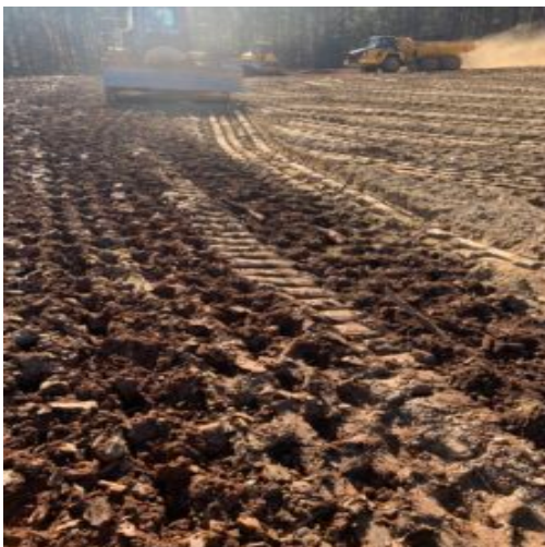
Fill placement at slope embankment ,topsoil and structural fill .
