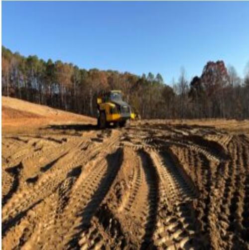
Slope area off road dump truck
