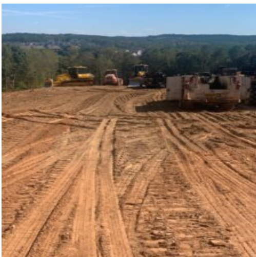
Sub grade prep at lots 72 & 73
