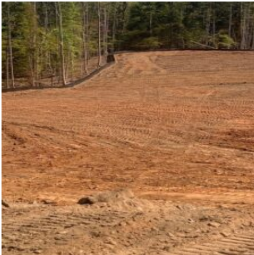
Existing graded areas
