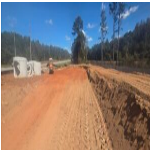
roadway in front of retaining wall
