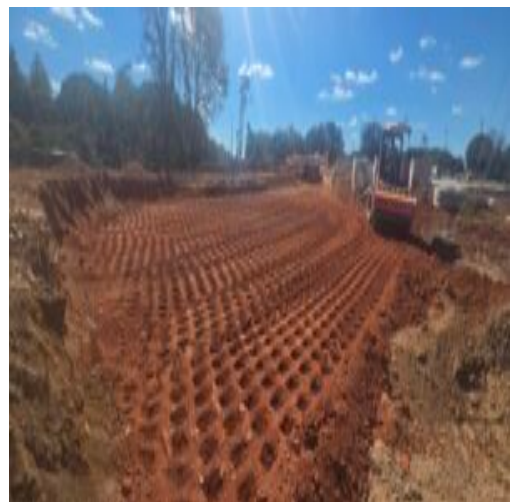
roadway in front of retaining wall
