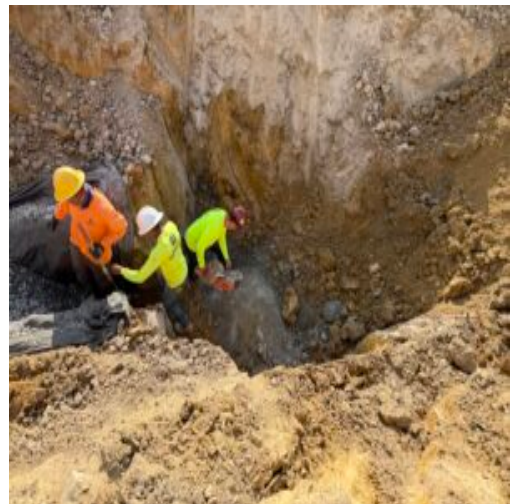
Manually cutting rock
