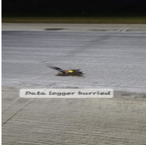
Picture depicting one of the data loggers buried in the concrete
