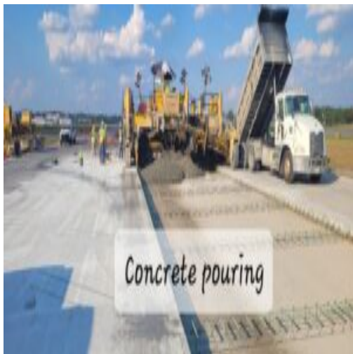
The concrete crews and the machineries
