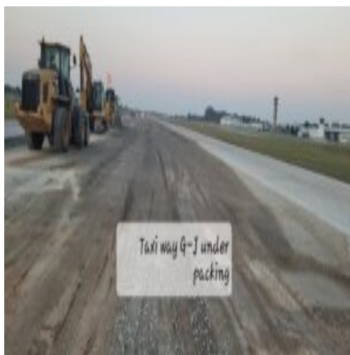
Picture depicting backfill and rolling of Taxi way G-J
