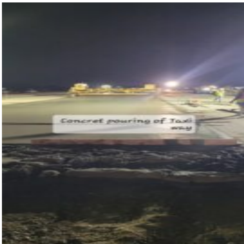
Picture depicting the entire pouring for the day
