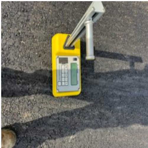
Density checks on in place binder mix
