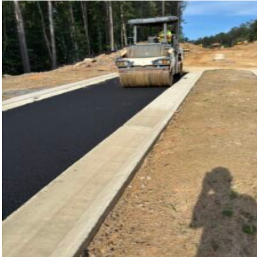
Compacting binder mix
