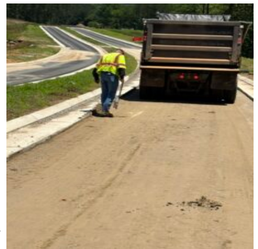
Proof rolling subbase stone at Nature Walk Pkwy. between sanitary sewer manholes #9 and 11 using a tandem dump truck with 19 tons.
