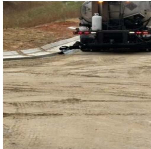
Tacking curb edges
