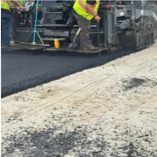
Paving at Phase 1B
