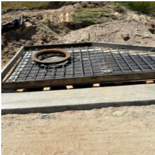
Observations of reinforcing steel at curb inlet throats
