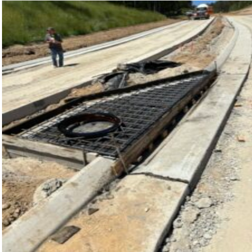
Observations of reinforcing steel at curb inlet throats
