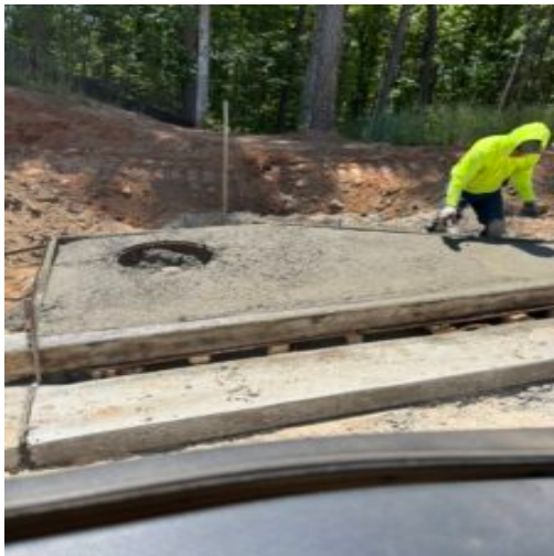
Pouring curb inlet throats
