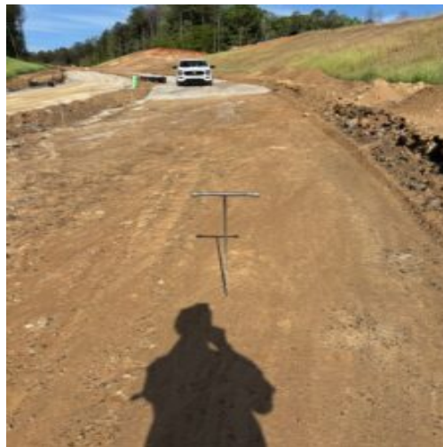
Sub grade approved for base stone placement
