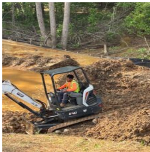
Repairing deficient area at toe of slope
