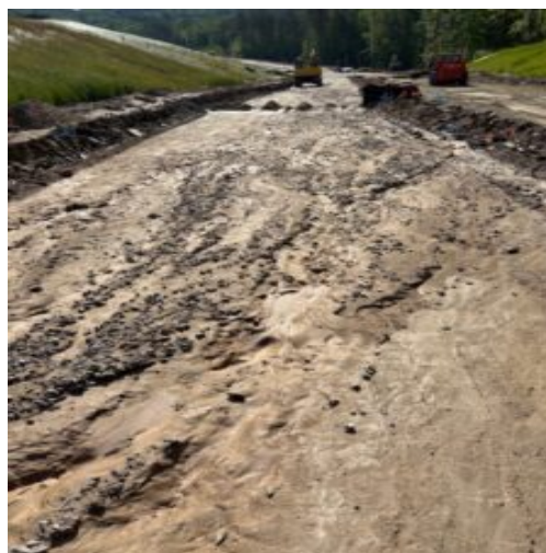
Approved area with rock in place
