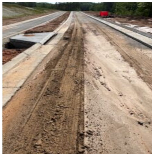
Washed silt over sub base stone
