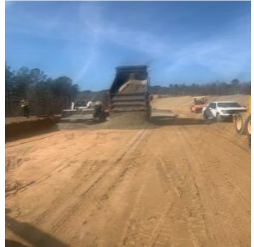
Back dumping rock to push over sub grade
