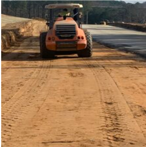
Compacting sub grade
