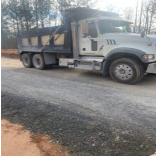
Observing loaded trucks with 18 tons backing across previous placed base stone
