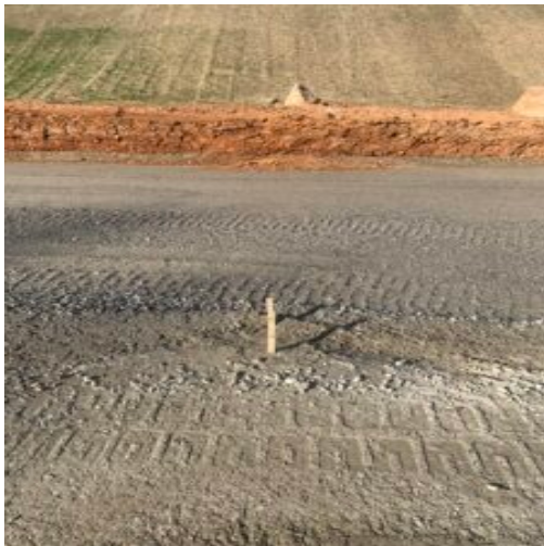
Grade stakes that were installed
