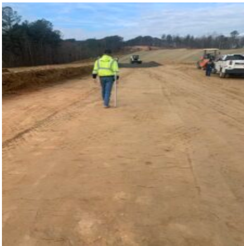
Observation of sub grade by Paving contractor
