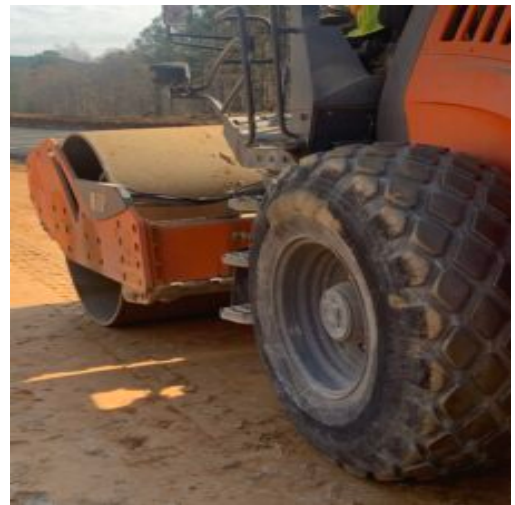
Sub grade prep. compacting using smooth
