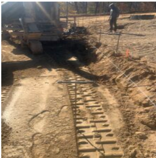
Curbing sub grade prep
