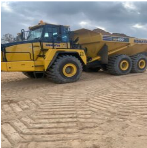
Proof rolling of sub grades at bldg. pads 1 thru 5
