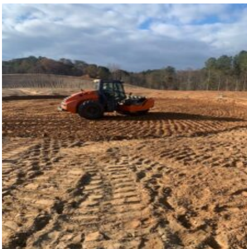
Sub grade prep. at cul de sac for curbing
