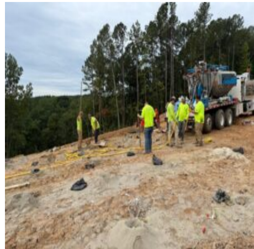
Preparation for blasting
