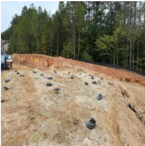
Preparation for blasting
