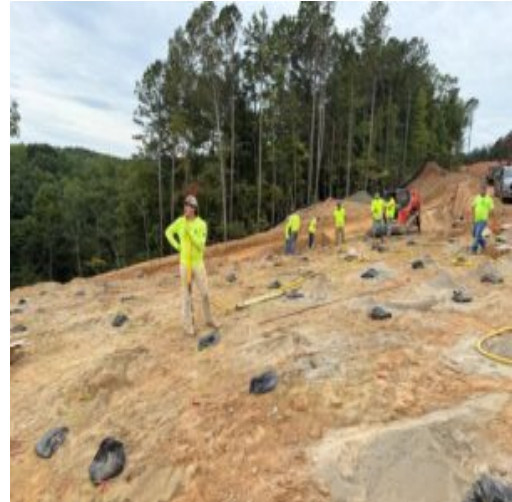
Preparation for blasting
