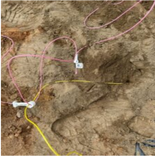
Preparation for blasting
