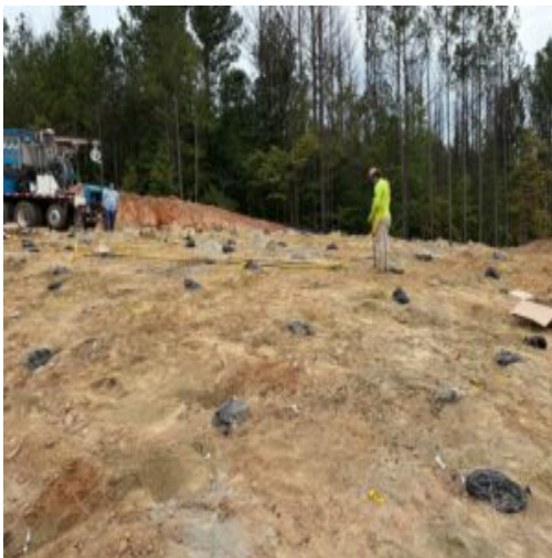
Preparation for blasting
