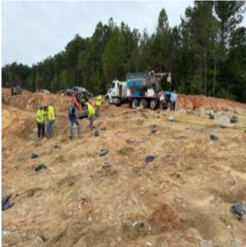
Preparation for blasting
