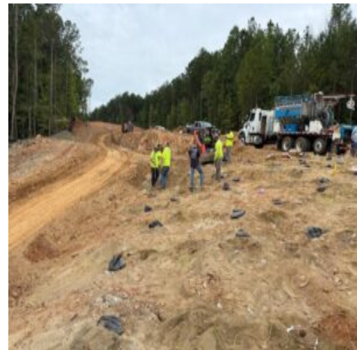
Preparation for blasting
