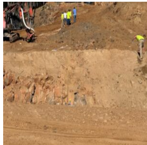
rock drilling in progress
