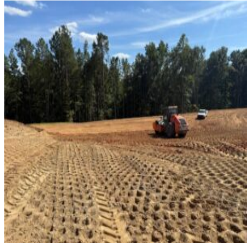
Backfilling in lots
