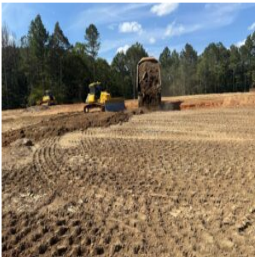
Backfilling in lots
