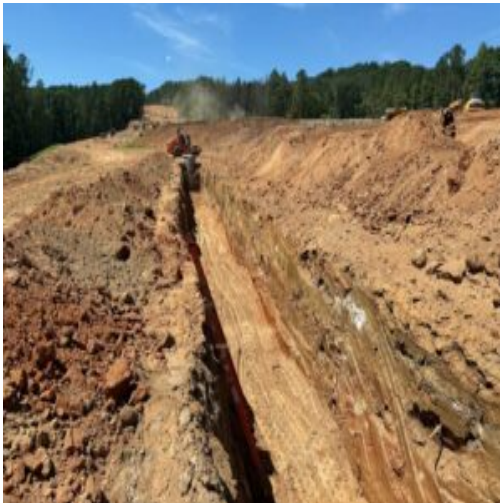
sewer line excavation
