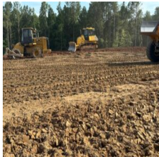
Backfilling in lots
