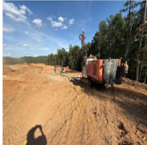
rock drilling in progress
