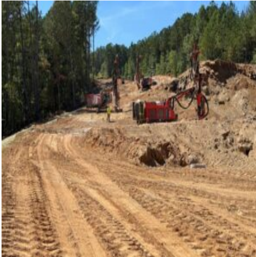
rock drilling in progress
