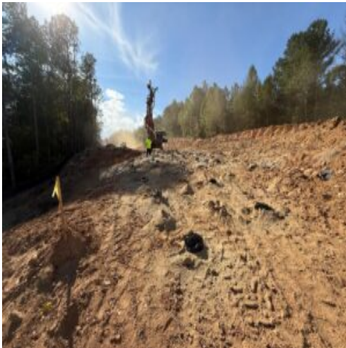
rock drilling in progress
