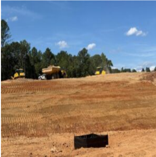
Backfilling in lots
