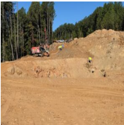
rock drilling in progress
