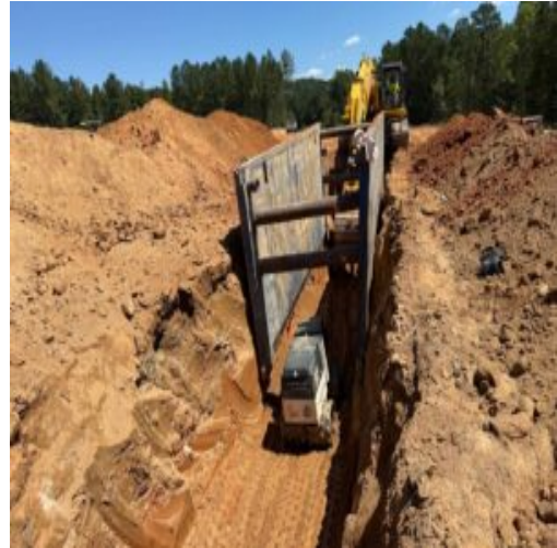
sewer line excavation
