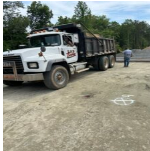
Proof rolling sub base stone with acceptable observations
