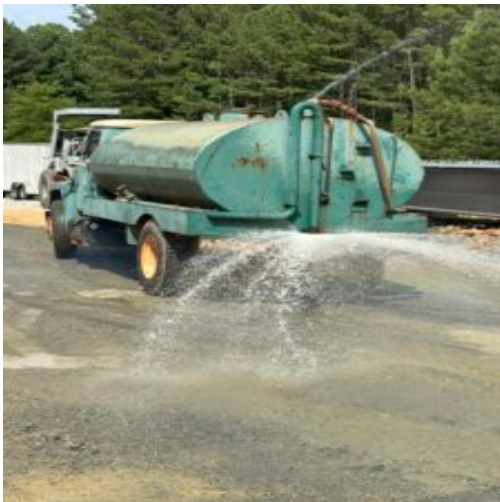
Placing water on sub base stone
