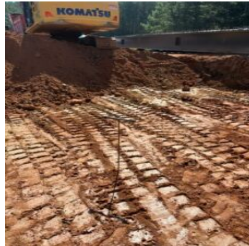
Observe sub grade by probing
