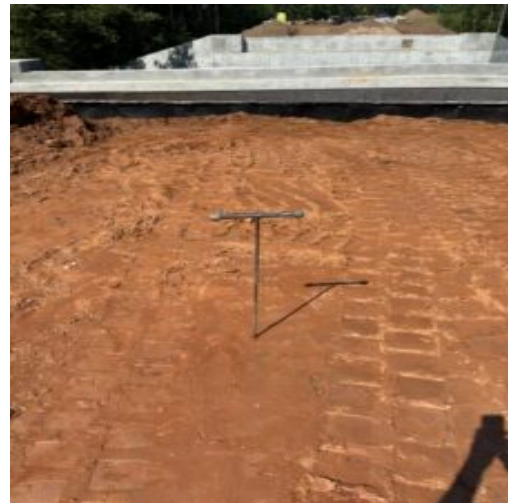
Observe sub grade by probing
