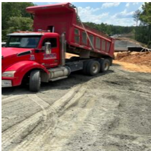
Placing GAB stone on approved sub grade soils
