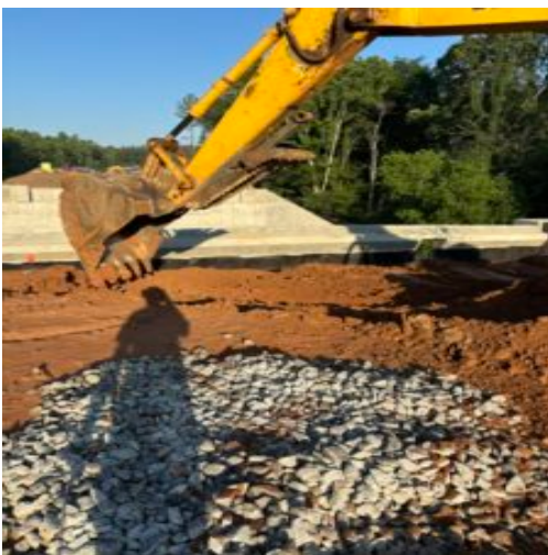
Begin sub grade excavation
