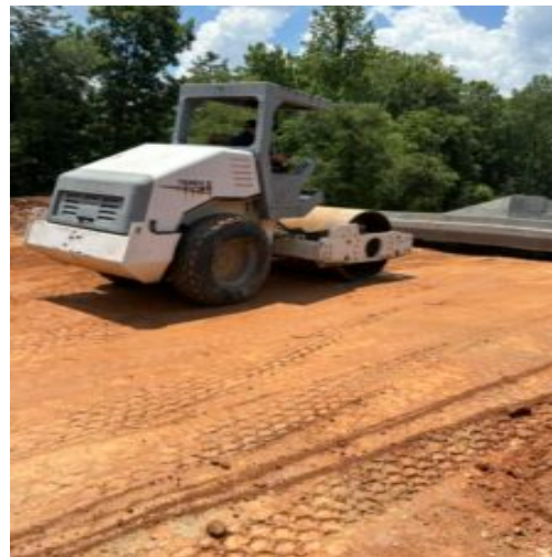
Compacting sub grade using vibratory smooth drum roller
