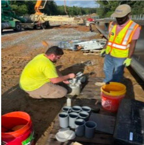
Performing air test
