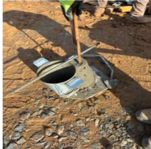
Performing slump test
