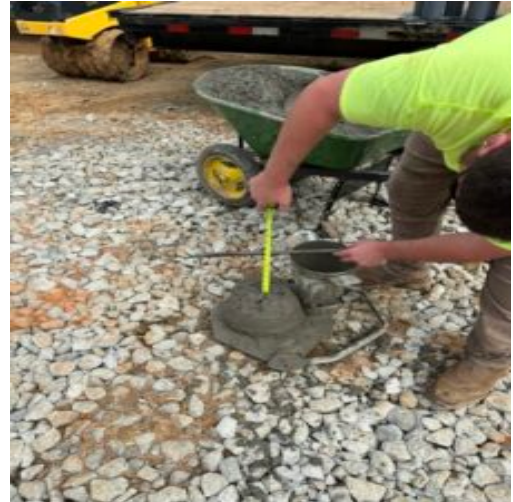
Performing slump test
