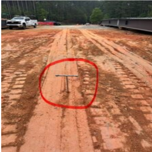
Recommended undercut area at crane pad
