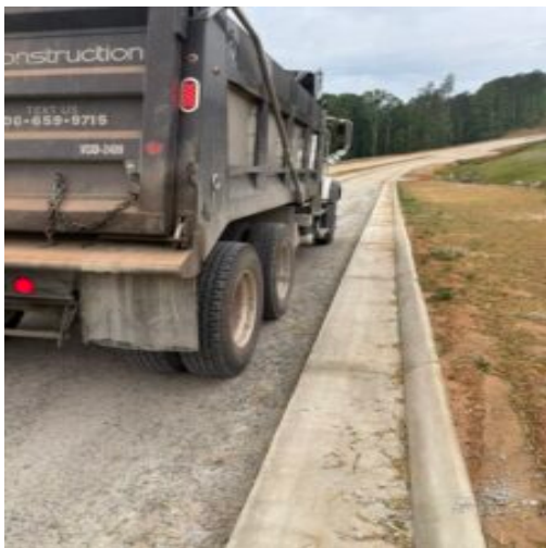
Proof rolling of sub base stone at Nature Walk Pkwy. between sanitary sewer manhole # 5 and 10 and drives to Phase 1A and 1B
