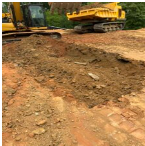
Undercutting crane pad
