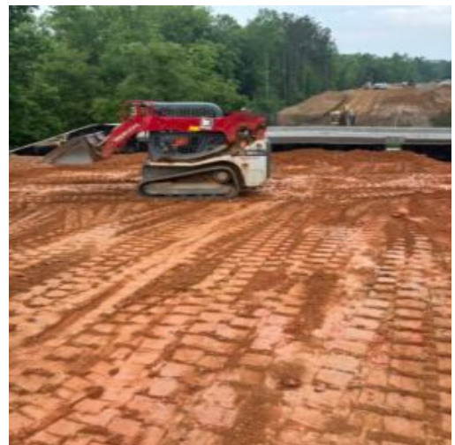
Placing fill at undercut crane pad.
