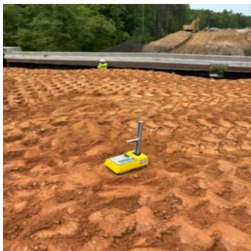
Performing density tests at wall backfill
