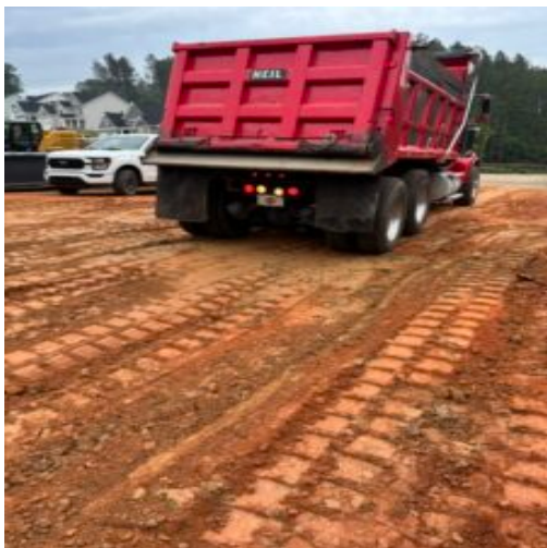
Proof rolling sub grade at crane pad to determine undercut
