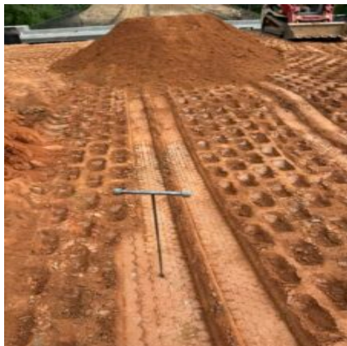
Observing backfill at undercut crane pad
