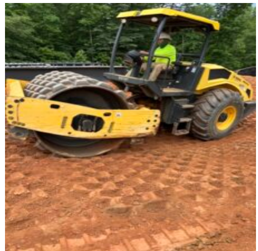
Compacting wall backfill
