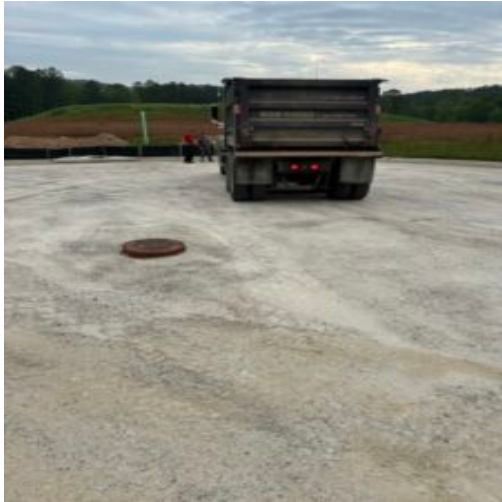
Proof rolling of sub base stone at Nature Walk Pkwy. between sanitary sewer manhole # 5 and 10 and drives to Phase 1A and 1B
