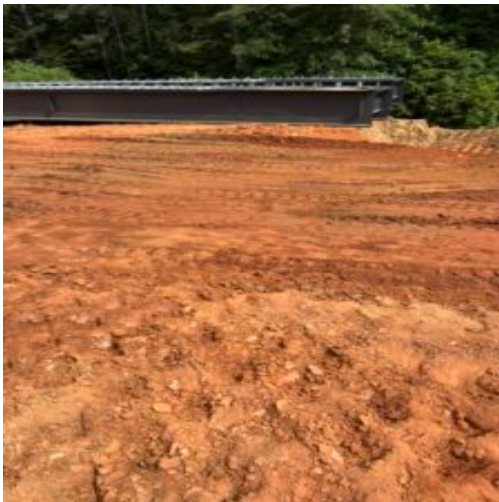
Fill placement and observation at north side bridge abutment. The compacting efforts were suitable for specifications.
