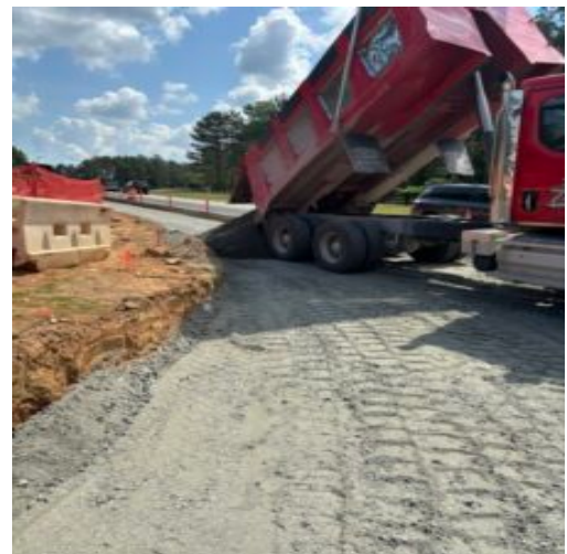
Subbase and sub grade observed at entrance to Seven Hills phase 13
