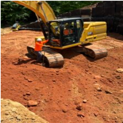
Placing and mixing onsite fill materials and performing density tests using a Troxler Nuclear gauge
