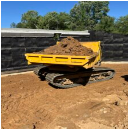
Fill placement and density tests at the bridge abutment.
