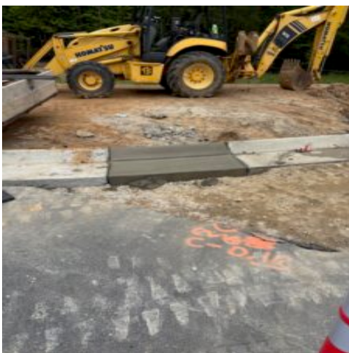
Poured throats at round about east side
