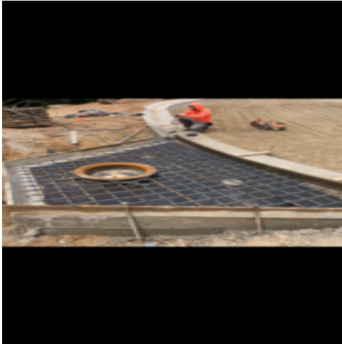
Reinforcing steel at throats
