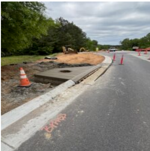
Poured throats at round about east side
