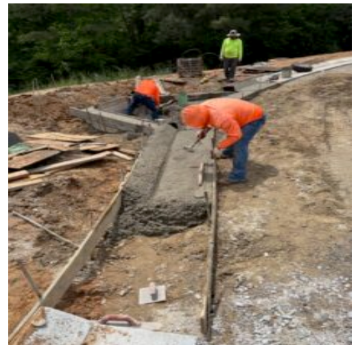
Pouring curbing and two throats at east side of round about.
