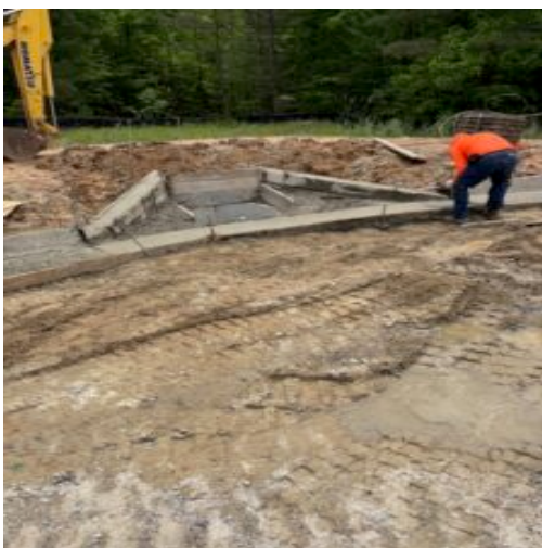
Pouring curbing and two throats at east side of round about.
