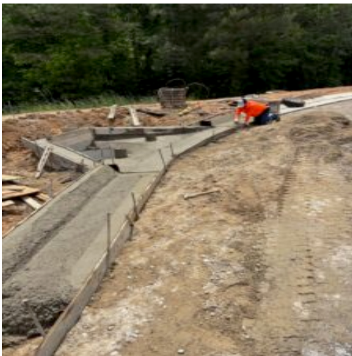
Pouring curbing and two throats at east side of round about.
