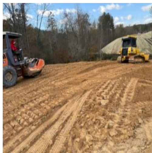
imported soil spread and compacted
