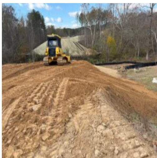
7 Hills BLVD side of future bridge
