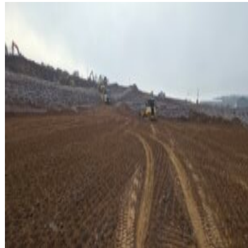
8 - 13 and 52 - 60 area, contractor removing pumping ground
