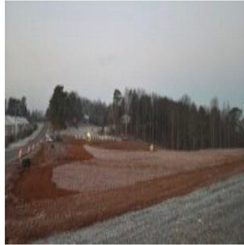
frozen ground being stripped
