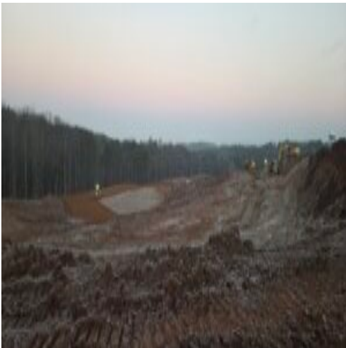
frozen ground being stripped
