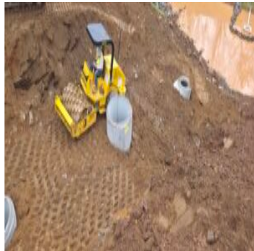
compaction around AA pipeline
