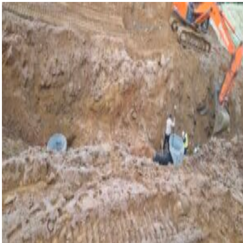
installing AA Pipeline
