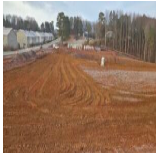
stripping frozen dirt
