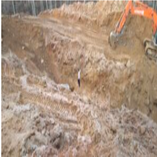
AA pipeline back detention pond area
