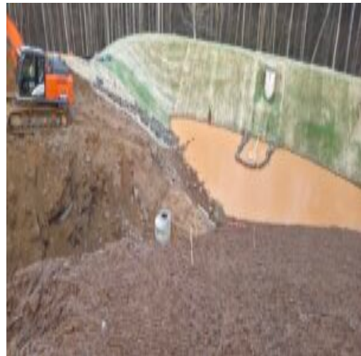
back detention pond area AA pipeline install
