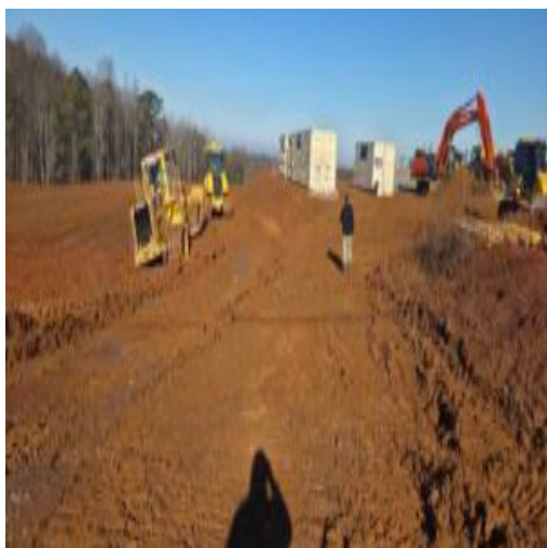
cutting mud/frost out before filling entrance way
