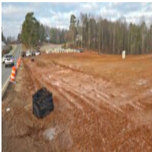
site conditions at beginning of day
