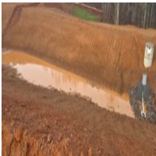
front detention pond
