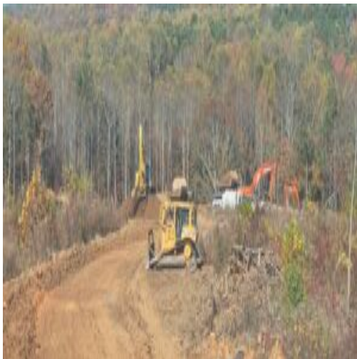
moving topsoil to pond
