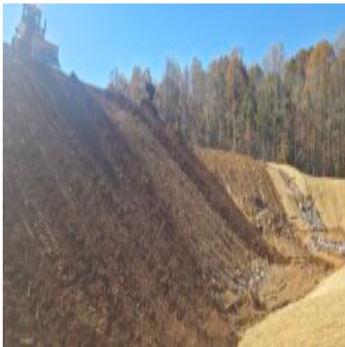
slope into pond
