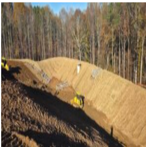
slope into pond
