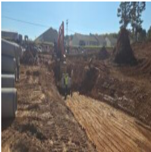
BC1 structure placement
