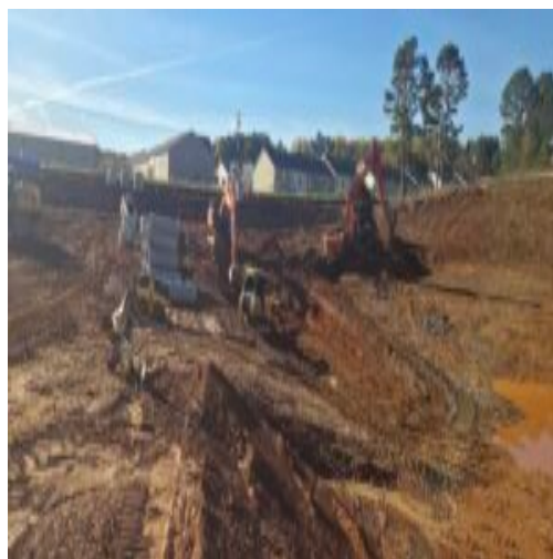
setting BC1 structure
