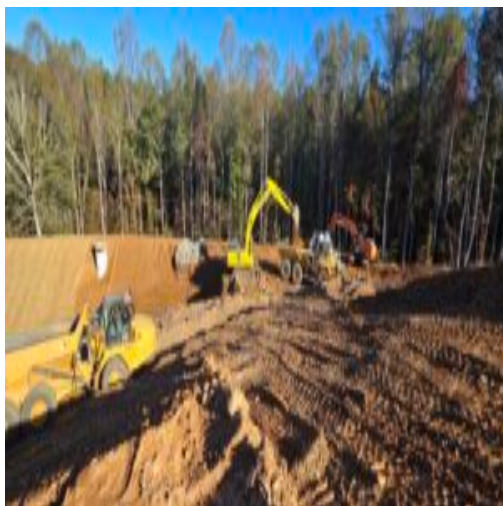
NW pond clean out
