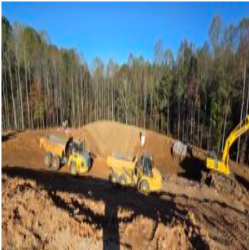
NW pond clean out
