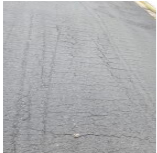
cracking
