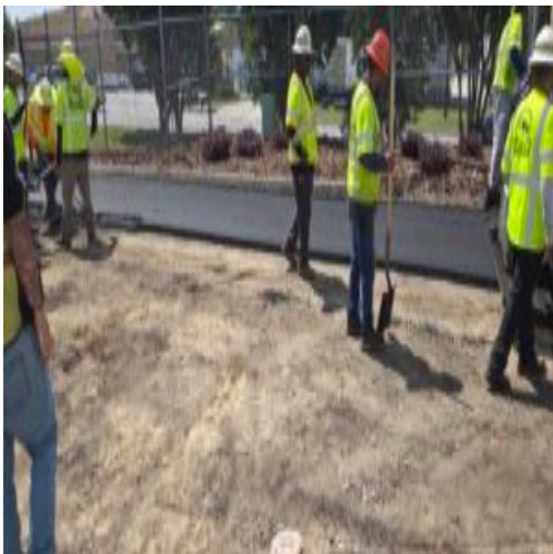
roadway behind hangar a
