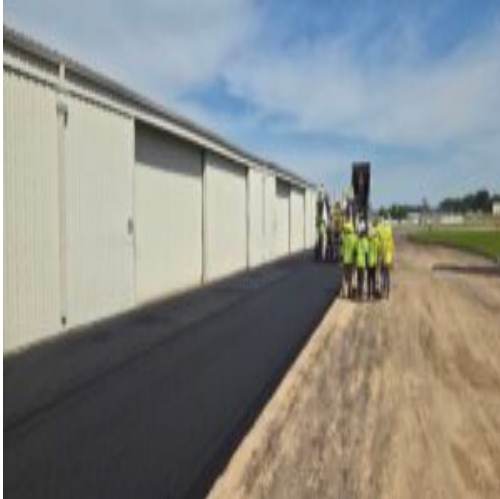
hangar a side
