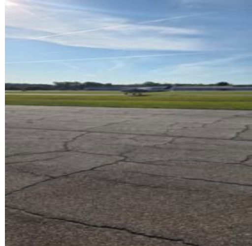
taxiway existing conditions
