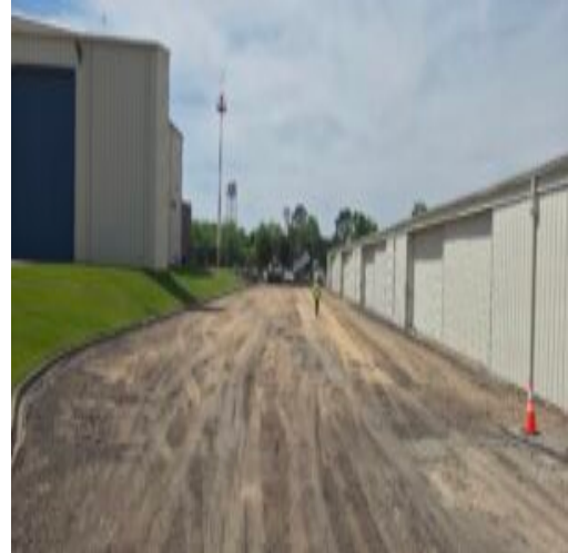
hangar a side
