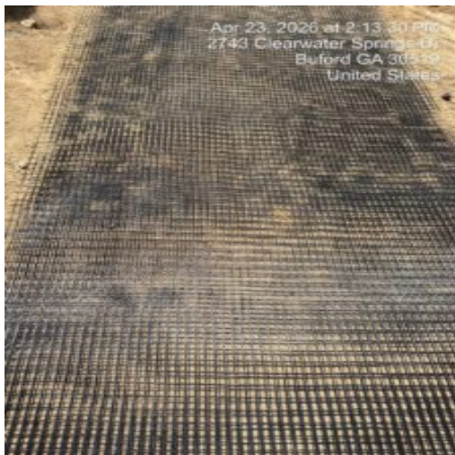
placing grid mat at wall 2
