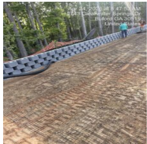
placing CMU blocks at wall 2
