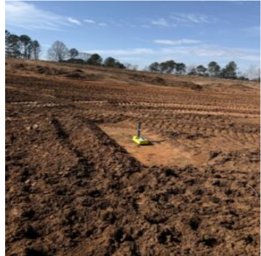
Density tests using Nuclear gauge
