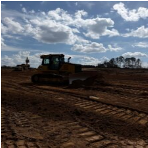
Spreading fill material using crawler bulldozer
