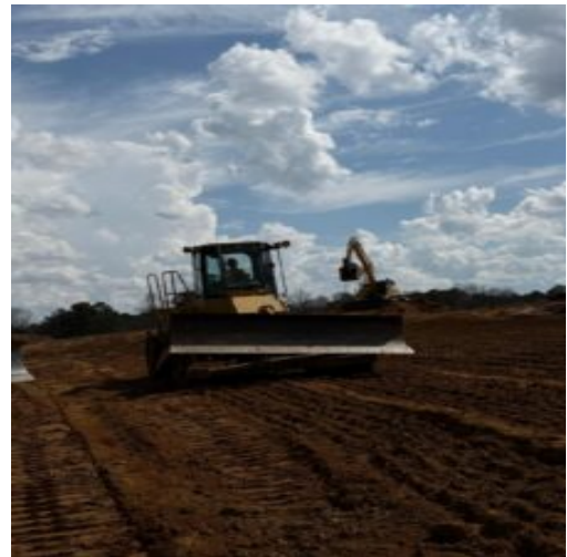
Compacting using pad foot roller 815
