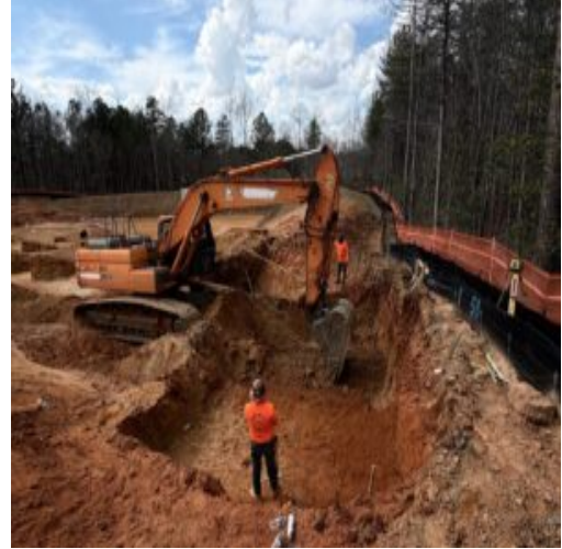
Levelling the subgrade for Concrete wall
