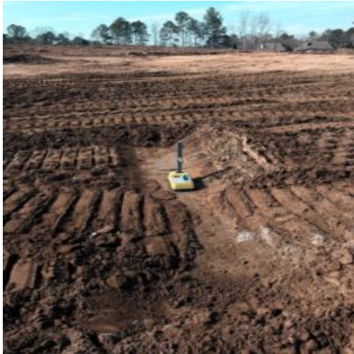
Density tests using Nuclear gauge
