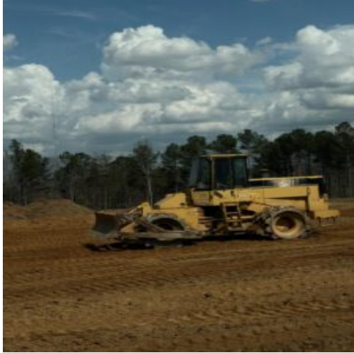
Compacting using pad foot roller 815
