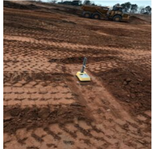
Density tests using Nuclear gauge
