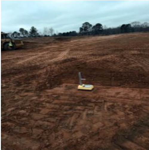
Density tests using Nuclear gauge
