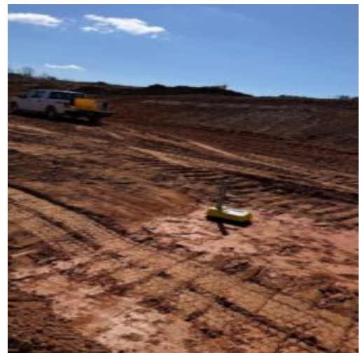
Density tests using Nuclear gauge
