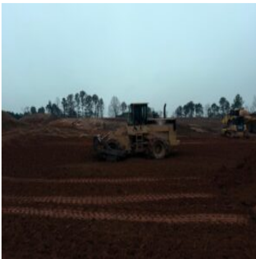
Compacting using 815 equipment
