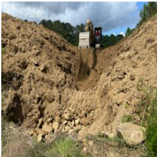
East looking west trench
