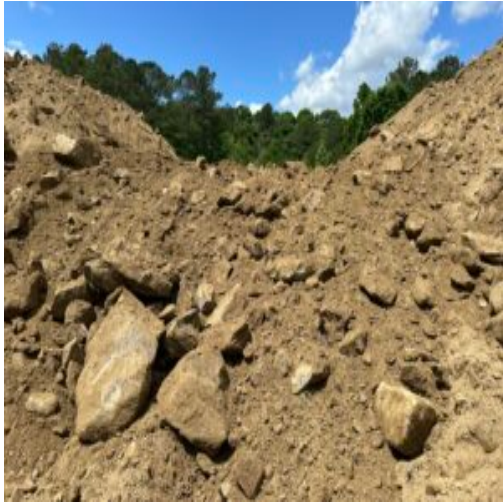
Trench refilled for safety.
