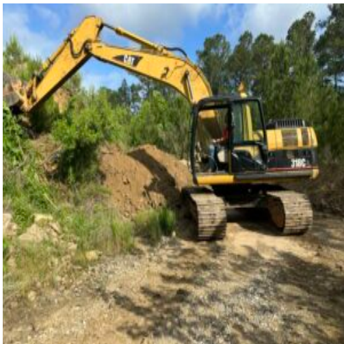
South west test pit
