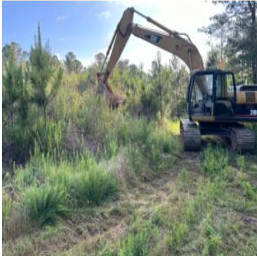
excavating south side
