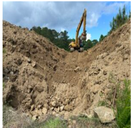
East looking west trench
