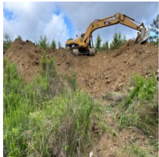
East to West trench
