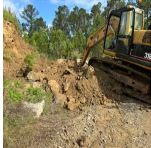
South West test pit
