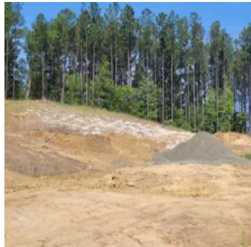
Entire area of blasting.
