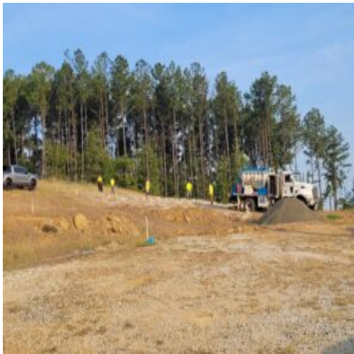
Several crew members putting explosives and connecting wires.
