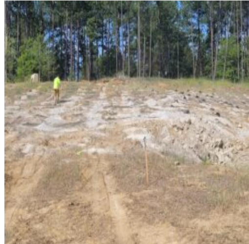
The guy confirming that exosives are put on all holes and wires are connected
