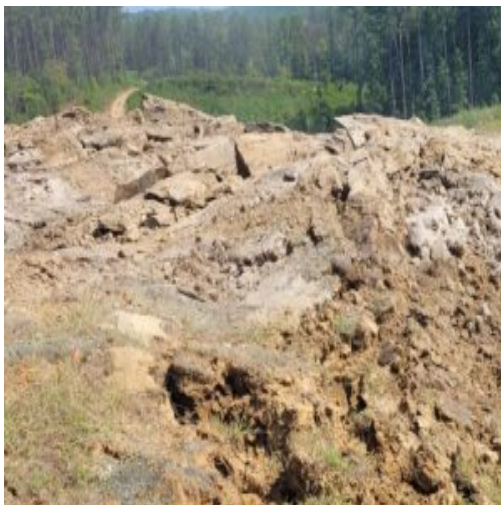
Site after blasting
