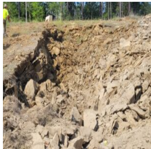
Picture depicting depth of blasting
