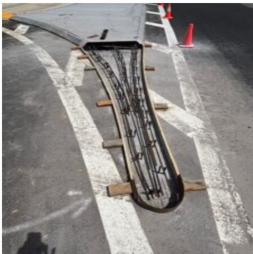
Added reinforcing #4 bars doubled in place of #5 bars.
