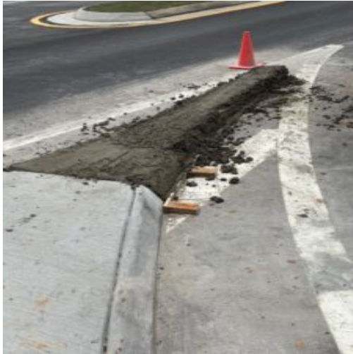
Pouring concrete at repaired area
