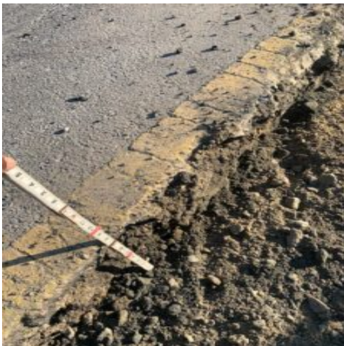
Removal and class B concrete placed at west side decel.island
