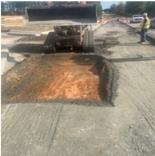
Two areas of subbase repair
