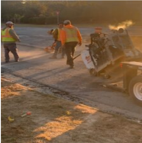
Saw cut and removal of existing asphalt at Seven Hills blvd,
