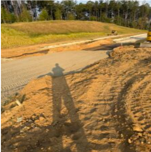
exit remediation area
