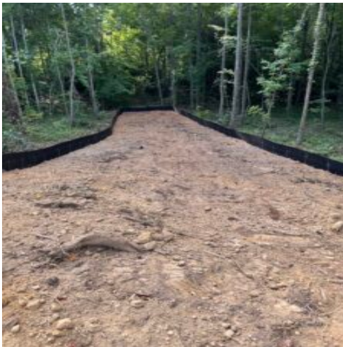
Section cleared containing 3 of the 4 future pier locations.
