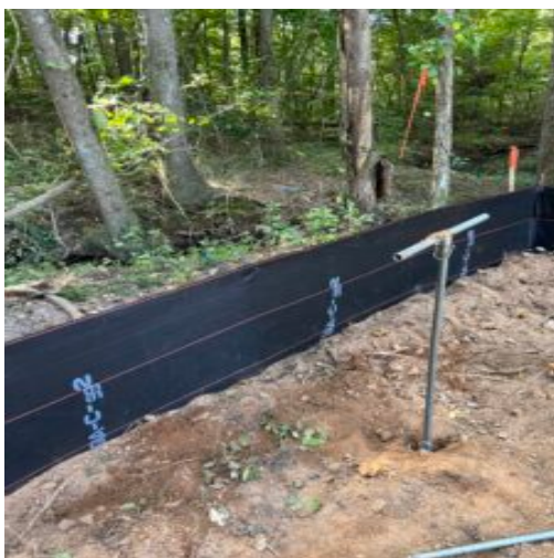
Location of Hole #4 is shown by auger inside silt fence, 5 feet from center of creek (and Pier location).
