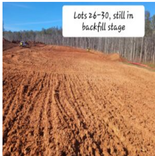
Picture showing entire backfill area
